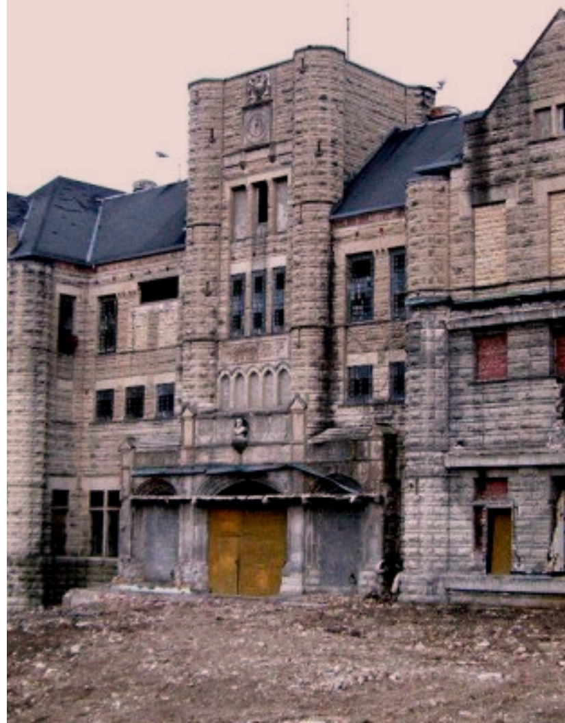
▼ Destruction to exterior penitentiary wall after tornado
