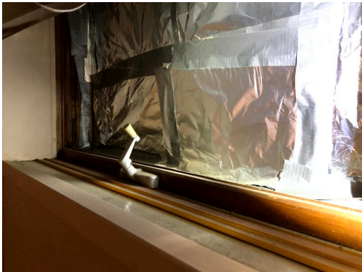
9. Windows in Dormitory
