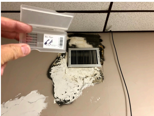
27. Stained Ceiling Panel - Location of Surface Sample 6I (Dormitory)
