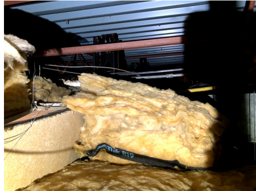
38. Above Ceiling Panels at Insulation and Metal Roof Decking
