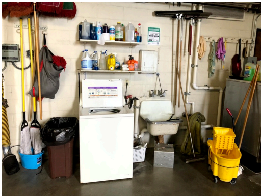
45. Laundry Area within Apparatus Bay
