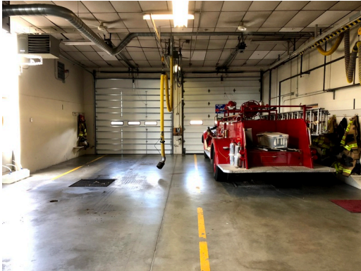
43. Apparatus Bay with Floor Drains
