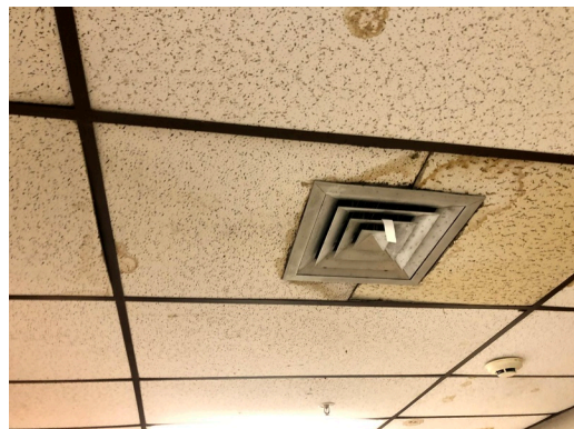
10. Stained Ceiling Panels and Damaged Plaster (Bedroom)
