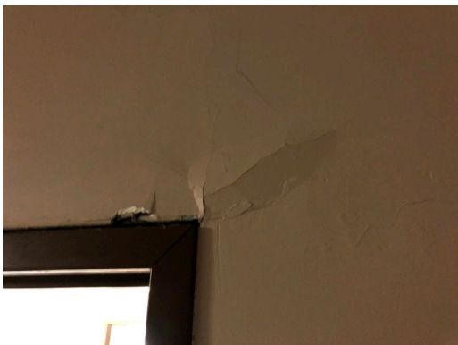
11. Damaged Plaster
