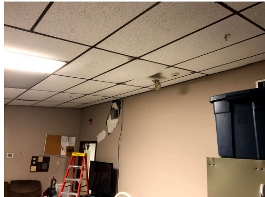
10. Stained Ceiling Panels and Damaged Plaster (Bedroom)
