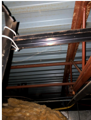
37. Above Ceiling Panels at Insulation and Metal Roof Decking
