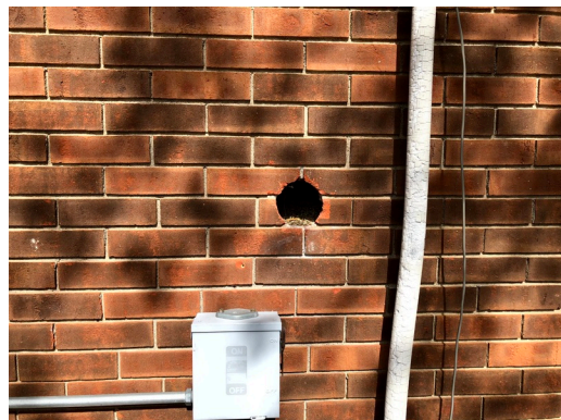
54. Location of former dryer vent
