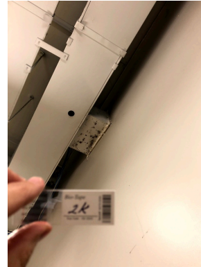
38. Hallway to Laundry Room - HVAC Ductwork - Location of Surface Same 2K
