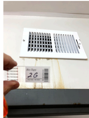
34. Bathroom (weight room) Stained Area - Location of Surface Sample 2G
