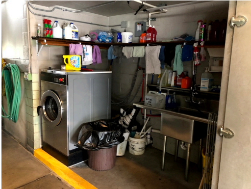
19. Laundry Area within Apparatus Bay
