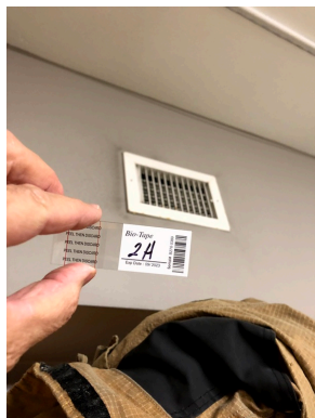
35. Dormitory HVAC Louver - Location of Surface Sample 2H
