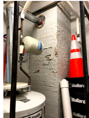
28. HVAC Room - damaged paint
