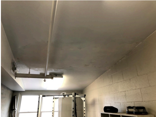
31. Weight Room - repaired ceiling
