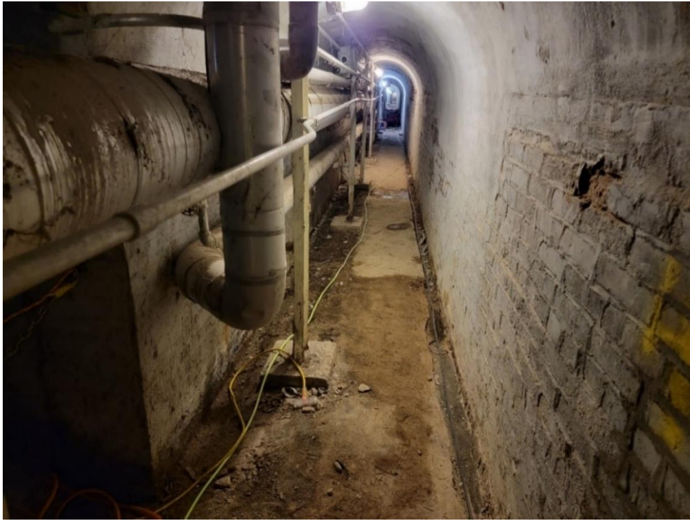
Figure 3-5: Steam Tunnel (Looking South from Feeder Tunnel Entrance)
