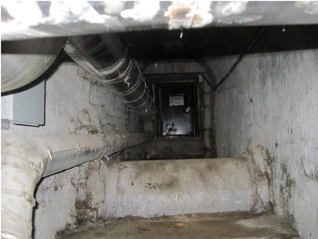
Figure 3-8: Pickard Hall Feeder Tunnel (View from the Steam Tunnel)
