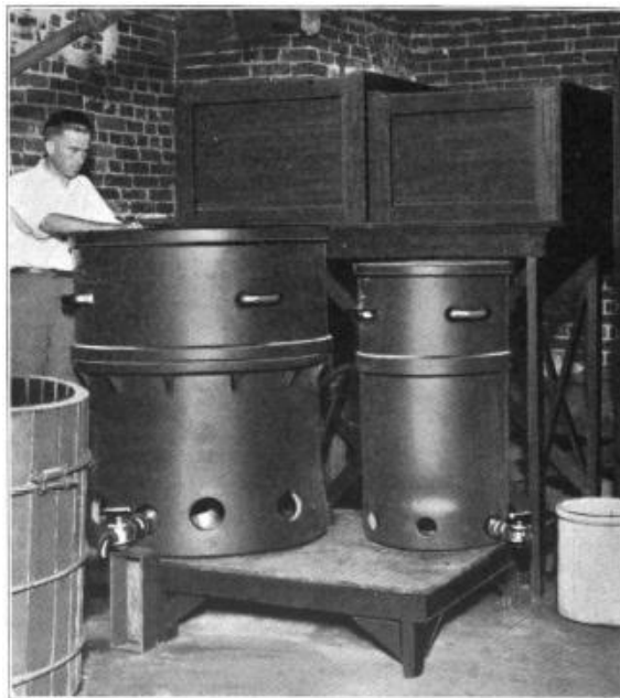
PLATE NO. 1. LEACHING POTS, BOXED, AND SUCTION FILTERS.
