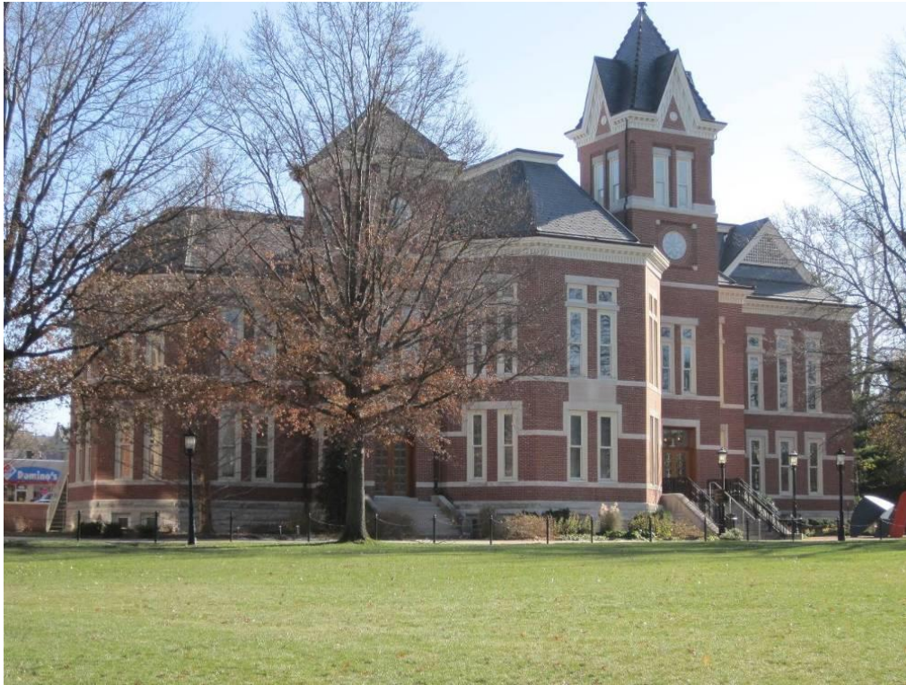
Figure 3-1: Pickard Hall – Looking Southeast
