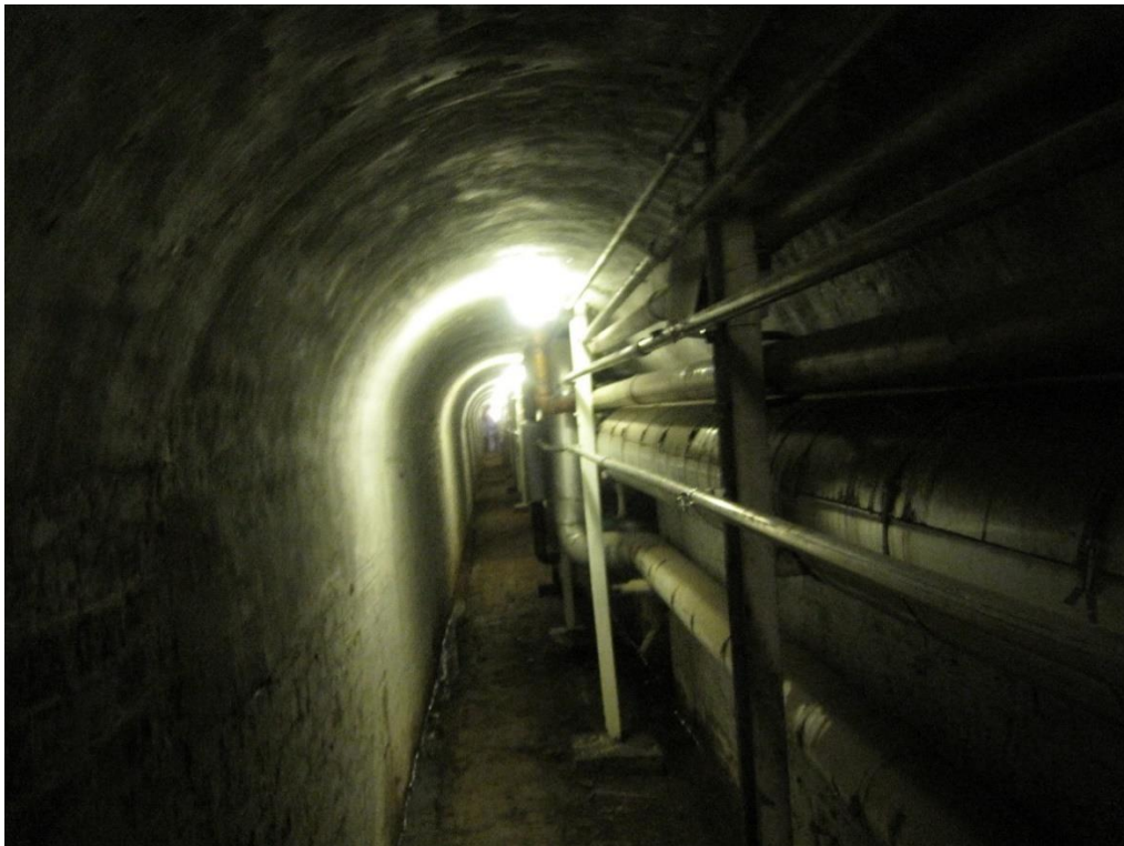
Figure 3-6: Steam Tunnel Interior (Looking North from Feeder Tunnel Entrance)
