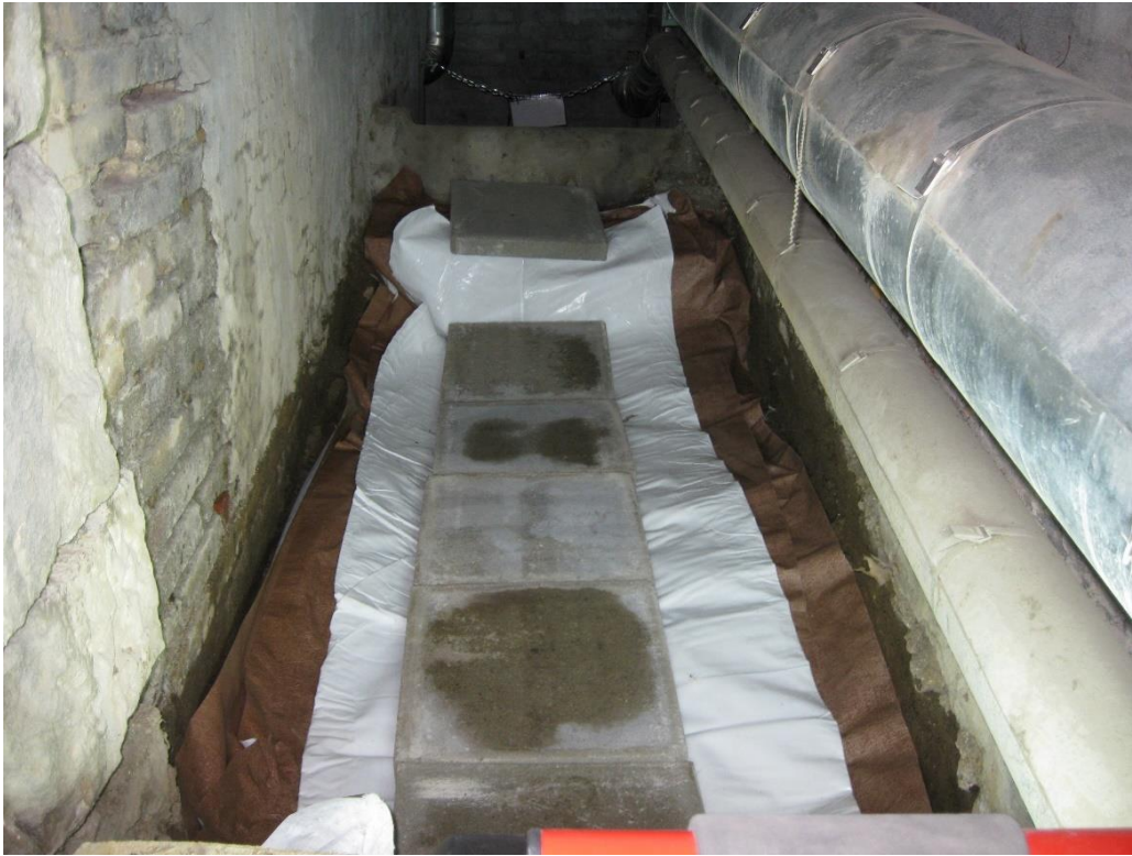
Figure 3-7: Pickard Hall Feeder Tunnel (View from Pickard Hall Room 15)
